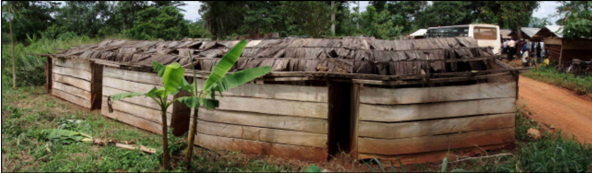
Figure 3.7: Unoccupied Speculative Structures at Amoma
