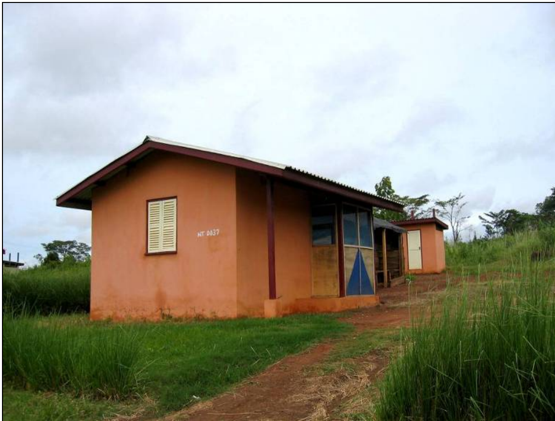
Figure 7.4: Typical House at the Ntotroso Resettlement Community
