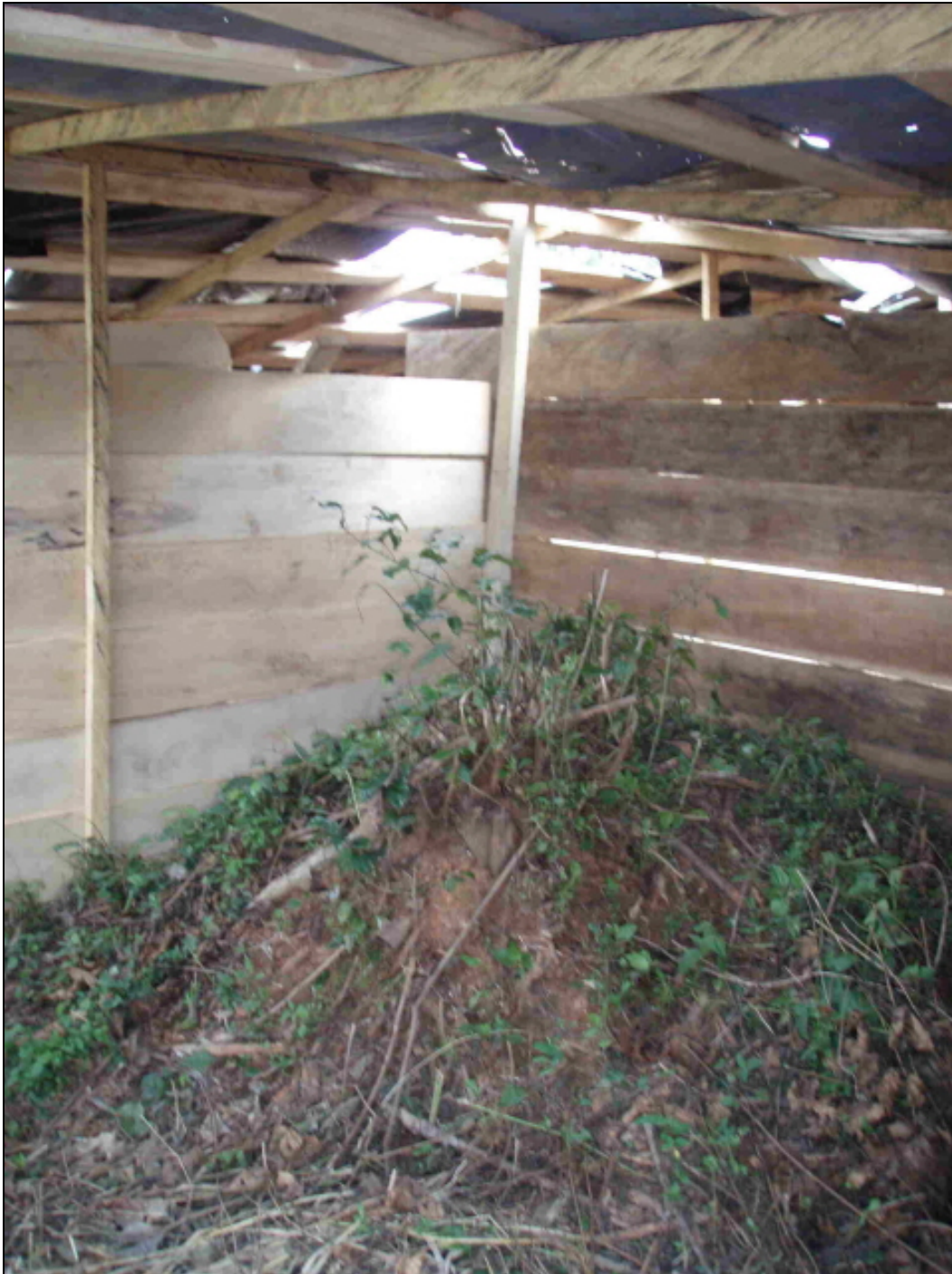
Figure 3.8: Interior of Speculative Structure (note tree stump)
